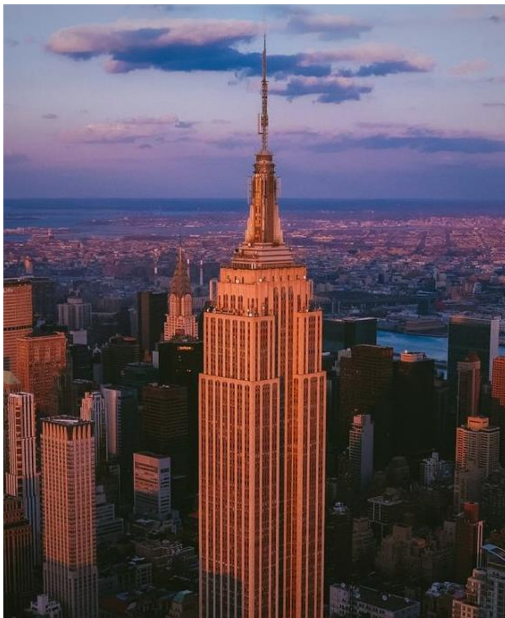
Slika 9. Empire State Building
