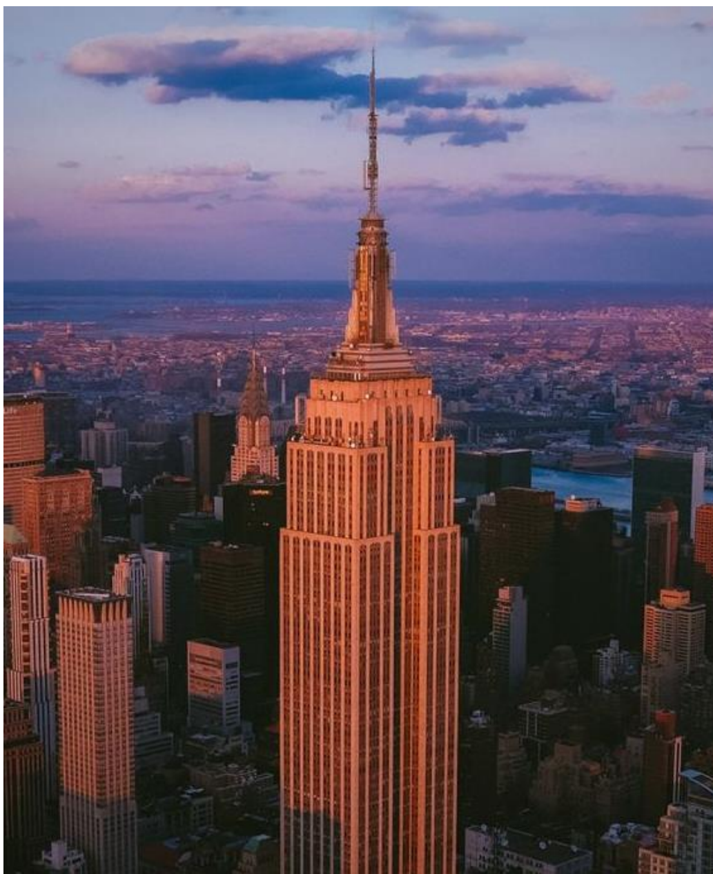
Slika 9. Empire State Building
