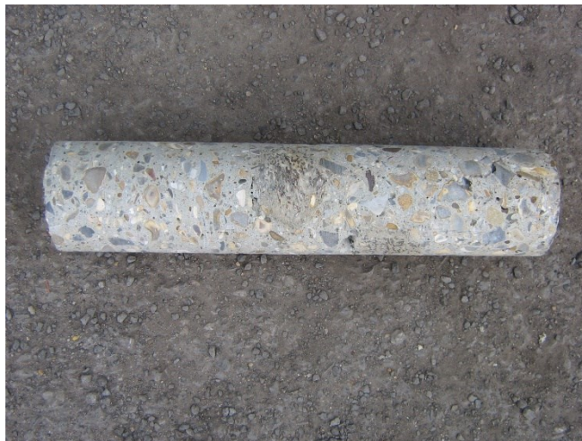
Figure 36: Concrete core sample taken for testing
