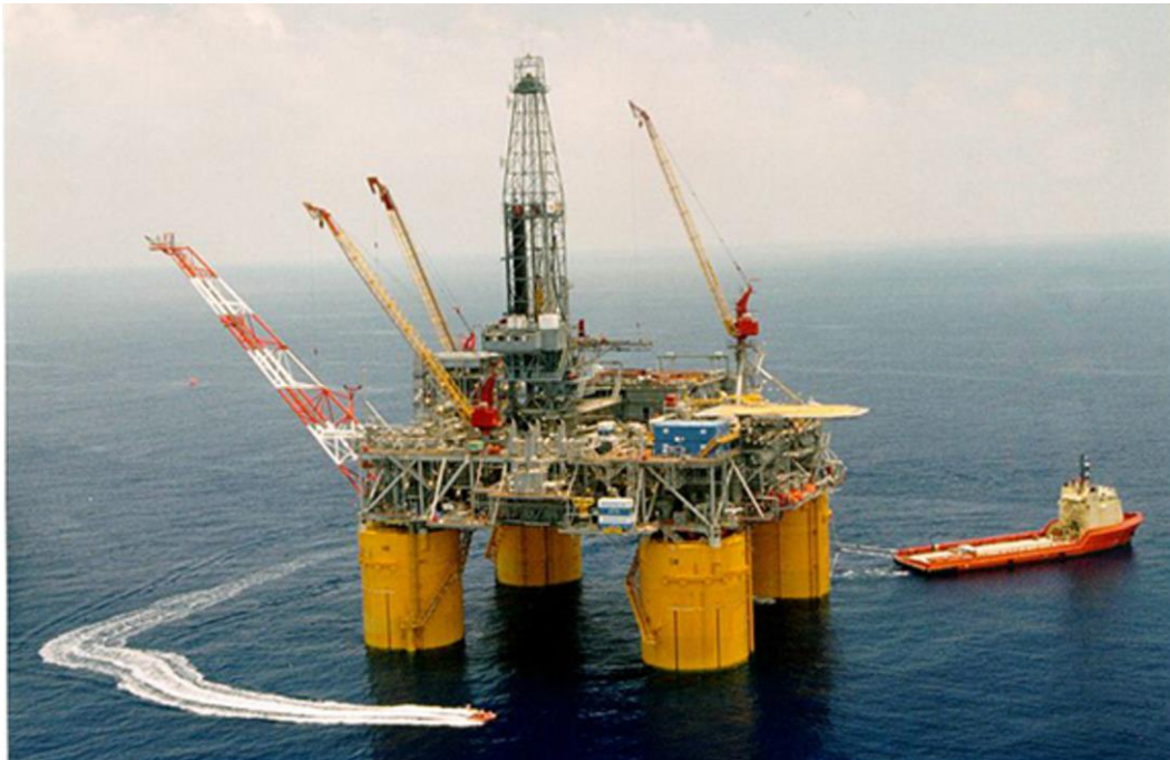
Slika 1.1 - Ursa TLP, nadvodni dio (Izvor: http://www.fastcompany.com/41051/life-board-gulf-mexico-oil-drilling-platform )
