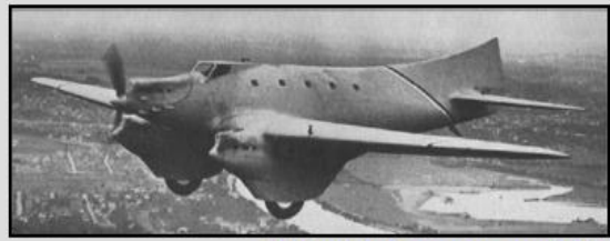
1932 : Wood structure and skins
