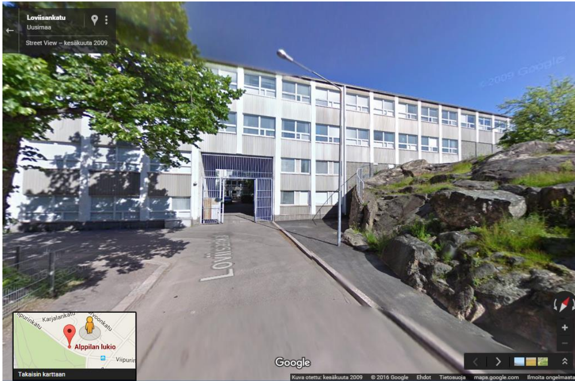
Figure 16 Google Street View representation of Alppila school building; Street View shows how the building profile is influenced by the shape of the rock slope
