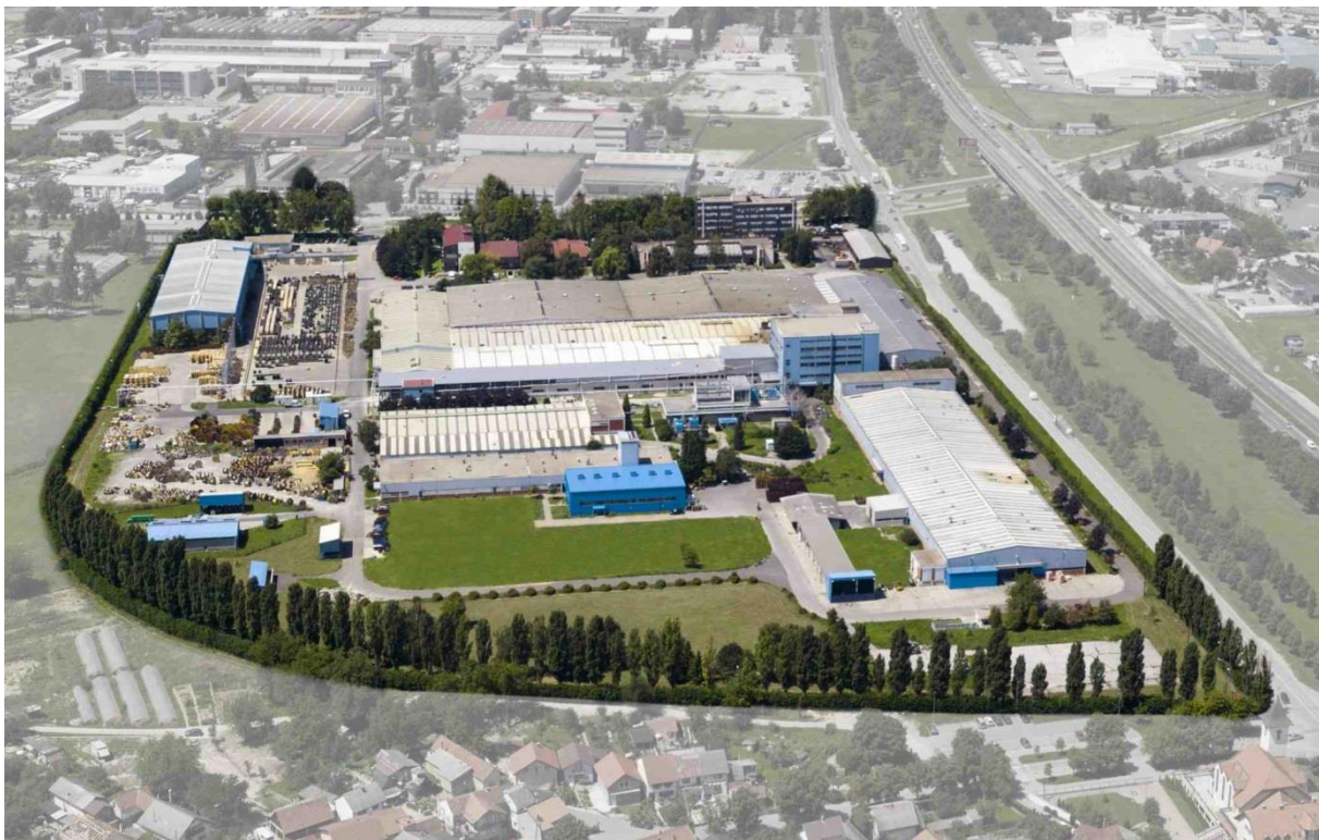
Figure 3-2 Top view of ELKA factory in Zagreb
