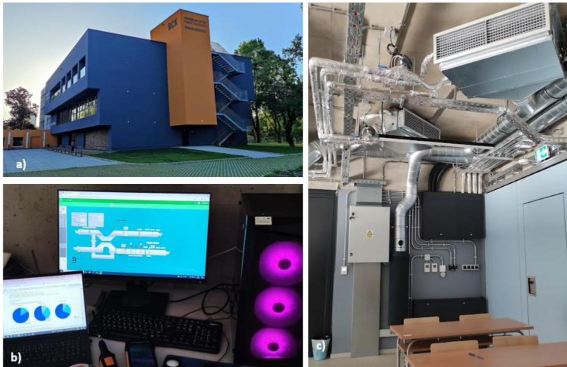
Figure 4.4 a) RCK Ruder Boskovic school building used as a living laboratory, b) SCADA system in the control room, c) various HVAC systems installed in the classroom that was used as a test bed
