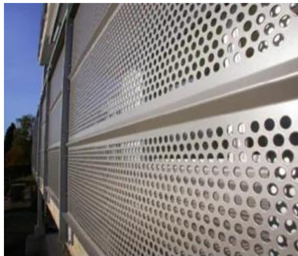
Figure 2.18 DSF system with perforated plates
