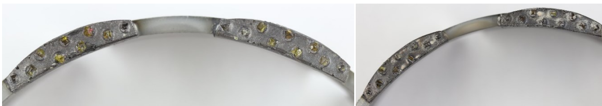
Figure 59: Close up photo of 2 segments on module #1 and #2
