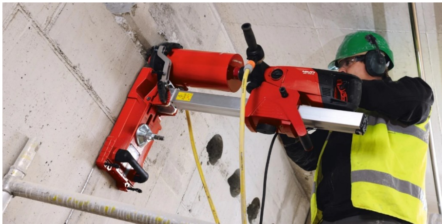
Figure 49: Hilti AG diamond coring system in application [24]
