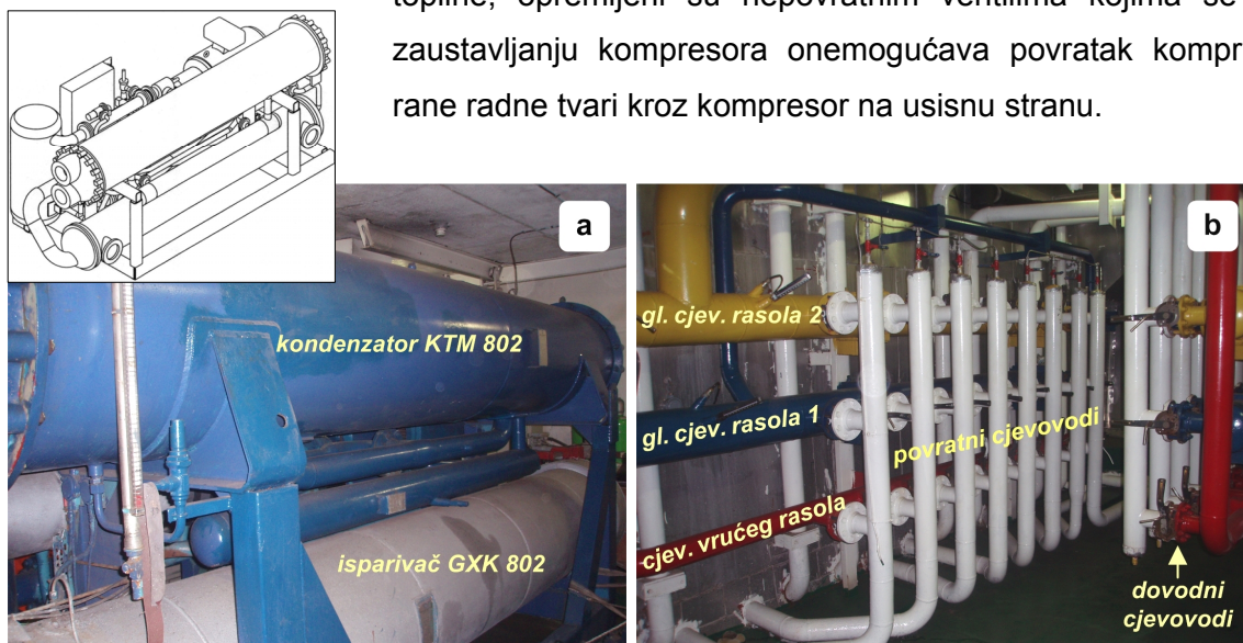
Sl. 2.14. Rashladnik rasola Sabroe Marine AB VSB 81E (a) i ventilske stanice rasola m/v "Lady Račišće" (b)
