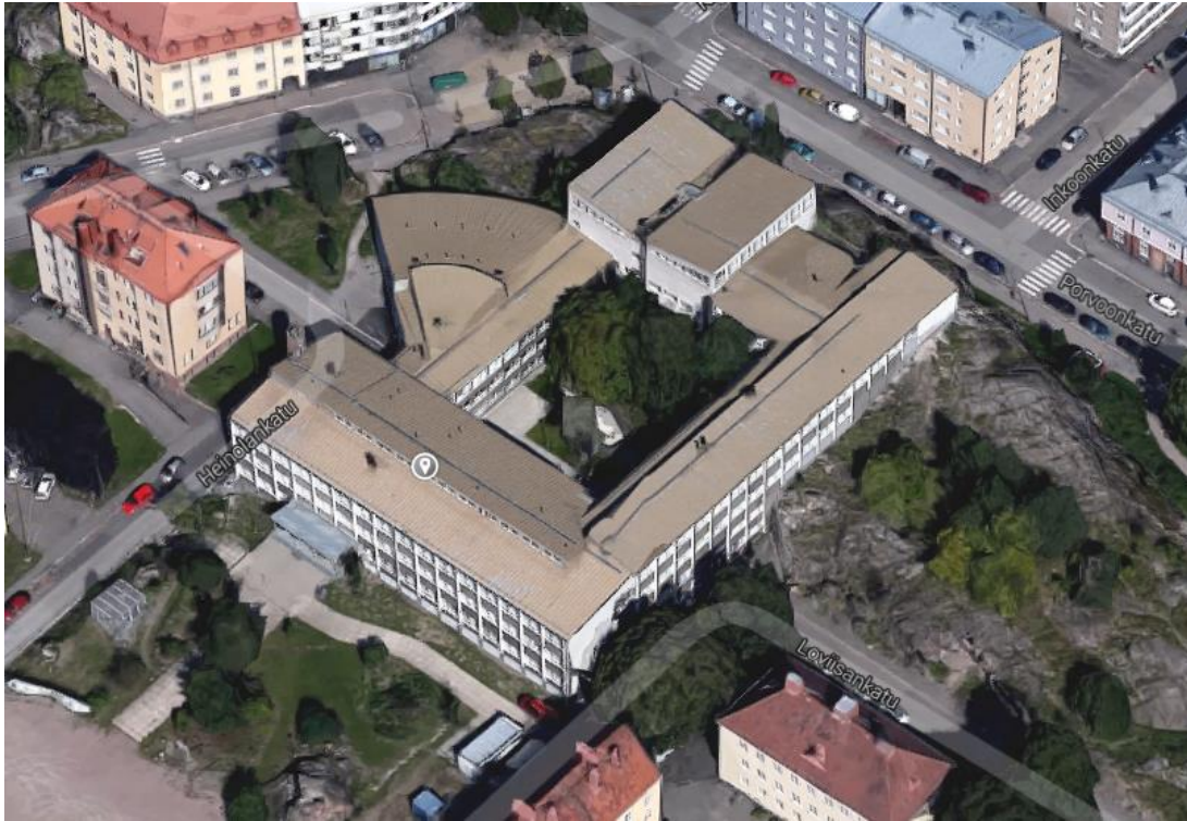
Figure 14 Alppila high school building located in Helsinki, Finland [31]
