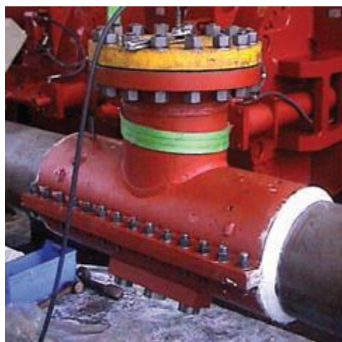
Slika 7.2 "Grouted tee" [52]
