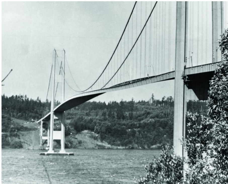
Figure 5: Tacoma Narrows Bridge flutter oscillations leading to a collapse.
