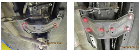
Figure 11: Improperly (left) and properly (right) fastened gearbox on the vehicle body.
