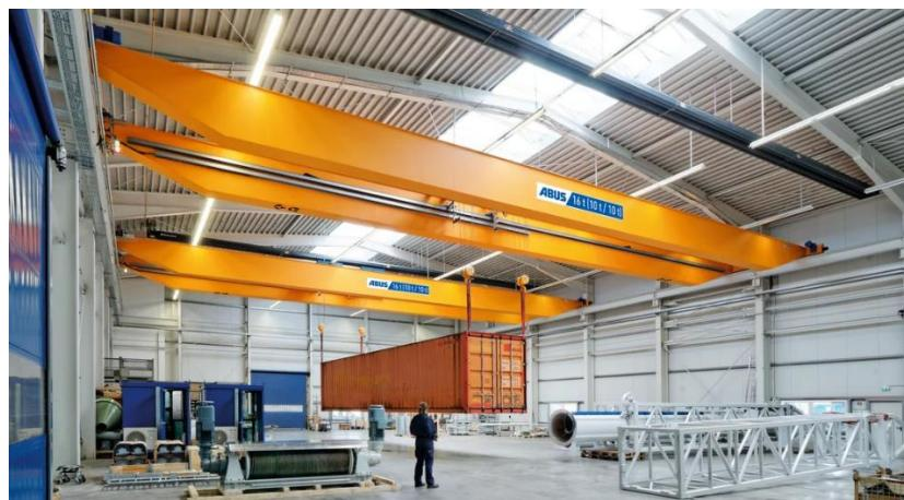
**Slika 4. Abus crane system – Double girder ovehead travelling crane**
